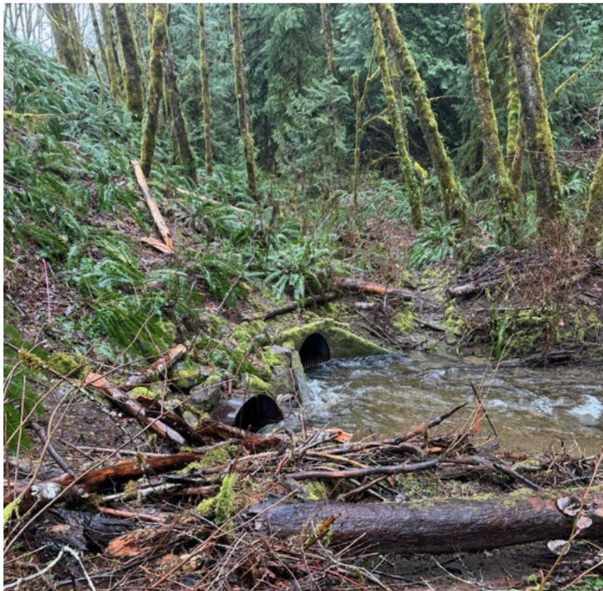
US Navy Railroad culverts are being improved for fish passage (current condition shown)
