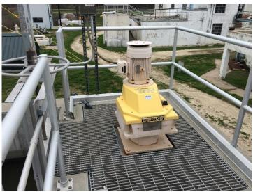
Currently, there are no operational issues with the raw water splitter box and rapid mixers. However, one of the rapid mixers is showing evidence of a bent shaft.
