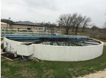
The mixer in Clarifier No. 2 is not operational. Without mixing energy in the reactionflocculation zone, more coagulant is necessary. The operators are currently feeding more coagulant yet are still seeing higher turbidities in the settled water as compared to Clarifier No. 1. This is evidence of inadequate flocculation energy or short-circuiting.
