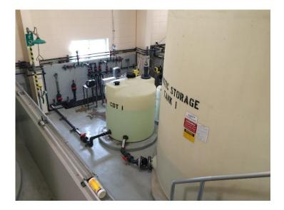
Photo 7. Chemical Tank and Piping
