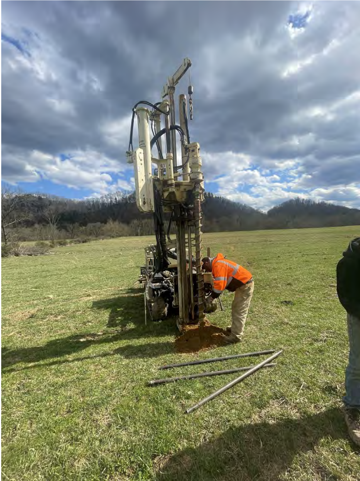
Figure 4: Boring activity on site; Cumberland River Industrial Park.
